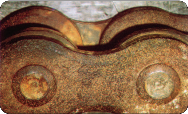
Figure 20 - Mode of Failure - Pitting Corrosion
