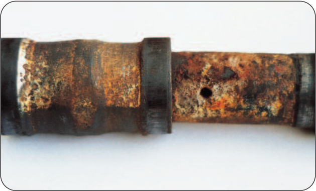
Figure 29 - Mode of Failure - Corrosion/Erosion
