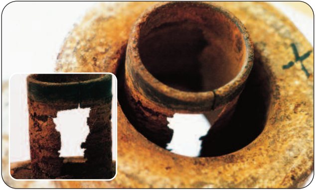
Figure 24 - Mode of Failure - Abrasion
